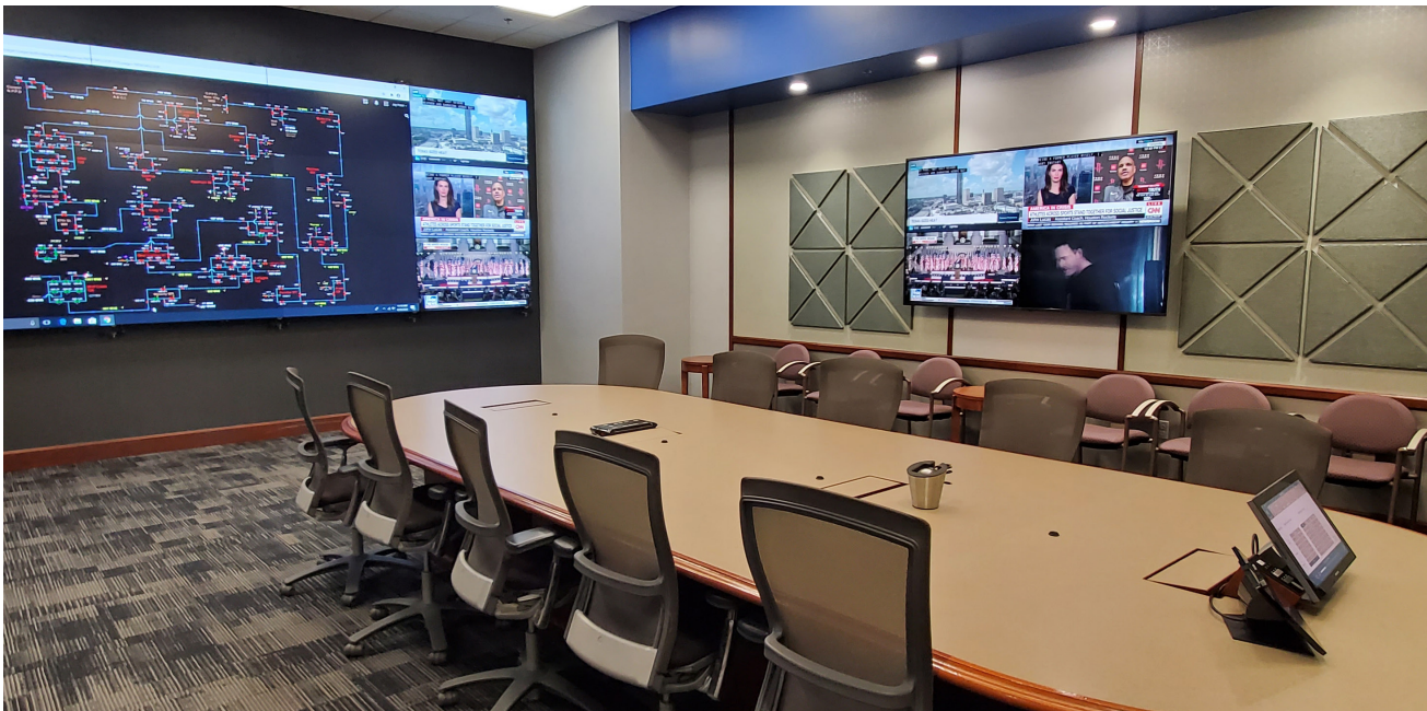
Twelve integrated 55-inch display panels make up the new display wall in Evergy’s Emergency Operations Center in Kansas City, Missouri.
